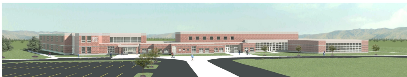
OVERALL FRONT VIEW
